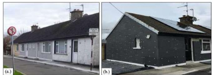
Figure 2. (a) Image of one block of terraces before retrofit [Source: SEAI] and (b) image of another block of terraces during retrofit [Source: 3CEA].
